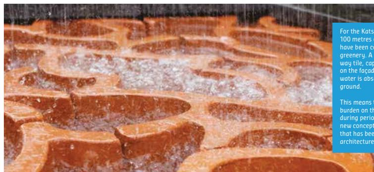
For the Katshoek Rain(a)way Garden, 100 metres of parking spaces have been converted into areas of greenery. A special tile, the Rain(a)way tile, captures excess rainwater on the façade and ensures that the water is absorbed slowly into the ground.
